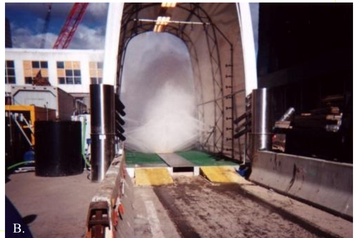
B. Waste water is collected and contained in channels below the mesh grating then disposed of in an environmentally safe manner.
